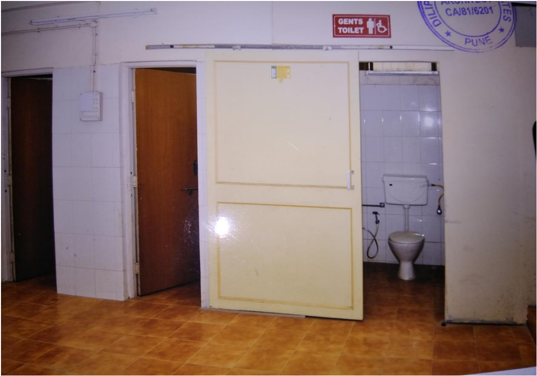
Gents Toilet for physically disabled
